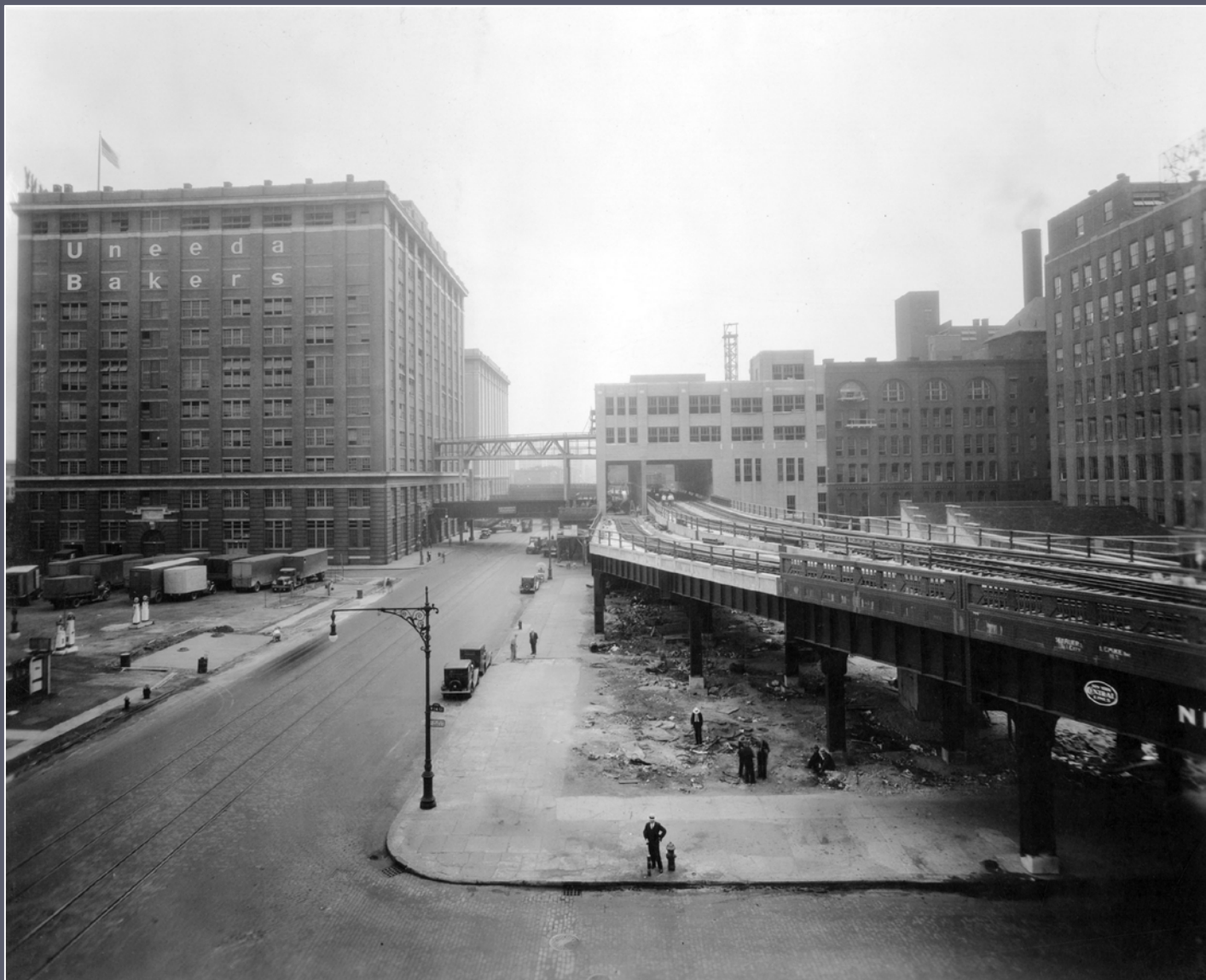
The High Line was an elevated freight train on Manhattan's lower west side, opened in 1934. It serviced the area's many industrial buildings, warehouses, meat packing district, shipping-related concerns, large-scale bakeries and other food-producing factories, and laboratories, such as Bell Labs. The tracks were not above the streets, but went right through the buildings.
