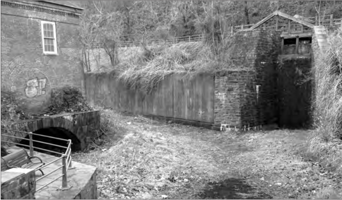
Figure 2. Remnants of the raceway system in Paterson (April, 2015). Note the sluiceway at the right which served to admit water from the upper canal at the top of the image. The circular pattern in the bricks on the wall of the industrial building on the left marks the former entrance of the rotating driveshaft. Photo: M. Kruge.
