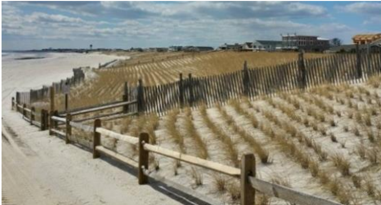
Figure 1.1 - Berm-dune construction Beach Haven, NJ.
