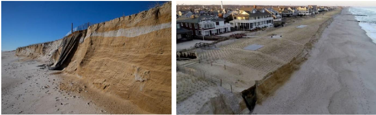
Figure 3.10 - Bay Head, NJ berm erosion and dune scarping (Doug Hood February 4, 2021 – Left and Mikes Davis & Thomas P. Costello February 5, 2021 – Right).
