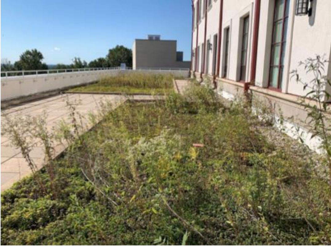
Figure 2. The extensive green roof has been incorporated on the CELS building on MSU campus. This is located on the third floor with two green roofs. Source: https://www.montclair.edu/facilities/sustainability/green-building-on-campus/
