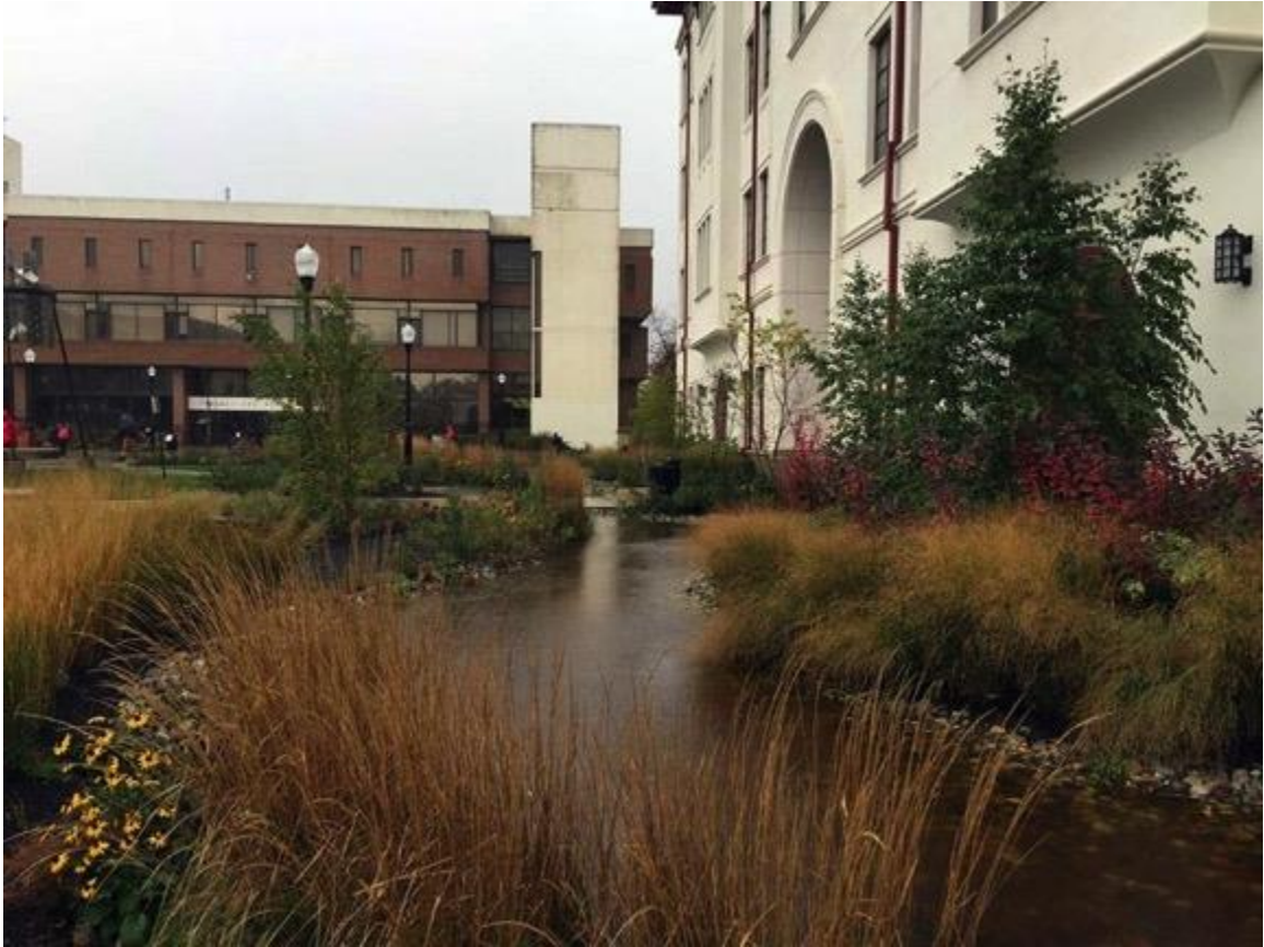
Figure 4. A rain garden design integrated in front of the CELS building. The stormwater runoff would be mitigated off the metal roofs and directed into the rain garden. Source: https://www.montclair.edu/facilities/sustainability/stormwater-on-campus/
