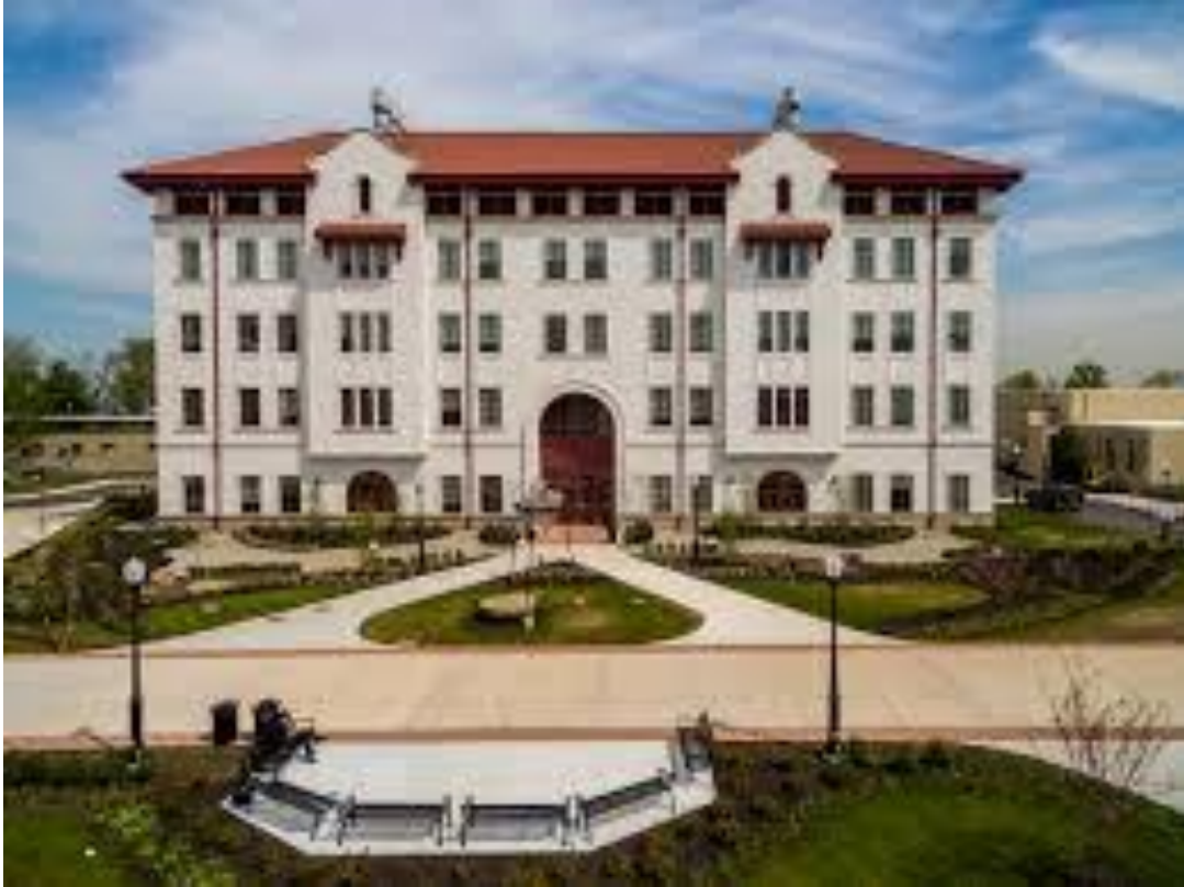
Figure 7. The bioswale application in front of the CELS building. The bioswale is connecting off from the sidewalks to reduce runoff. Source: https://www.usgbc.org/projects/cels
