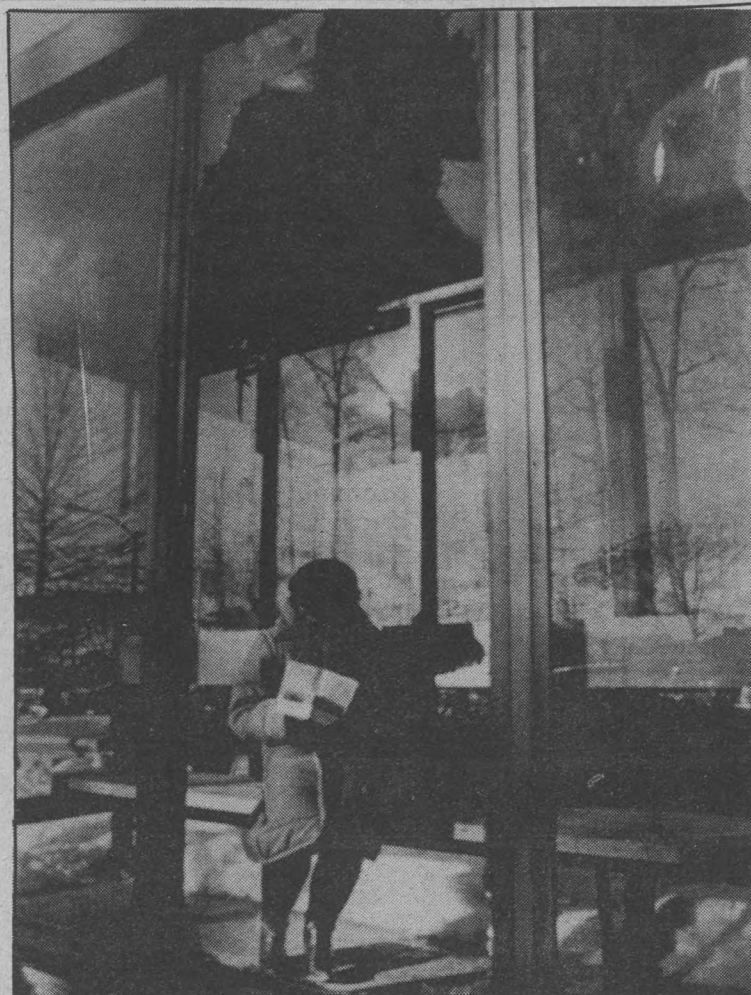
Icy conditions caused a snowplow to lose control and shatter the glass in the TNJ bus shelter this week.
